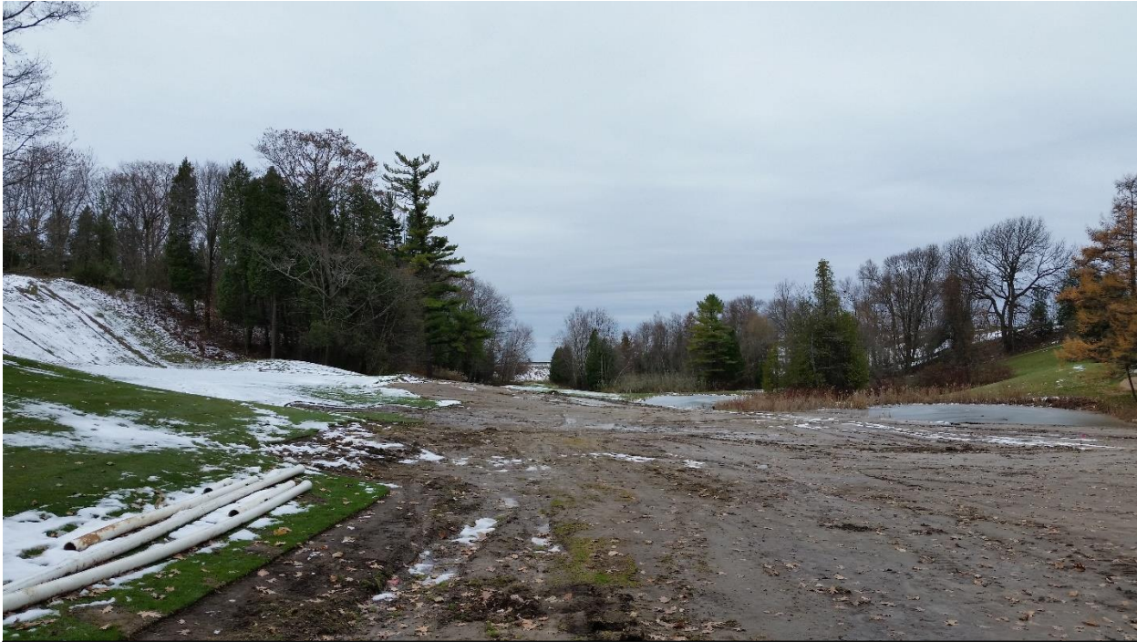
Port Hope Golf & Country Club: Hole No. 18 During Construction
